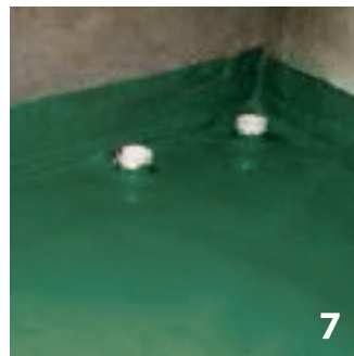
Completion of Obaproof AB Top Seal 119
